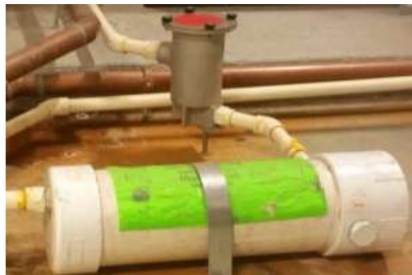
Figure 8-7: Condensate Trap and Neutralizer
